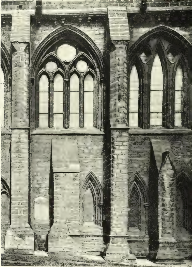
Exterior of second and third Bays east of Blacader's Aisle.
